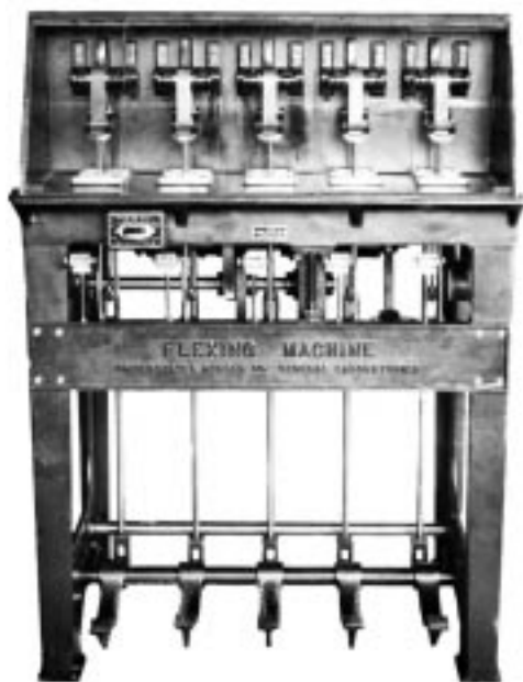
FIG. 1 Scott Flexing Machine with Five Hubs
